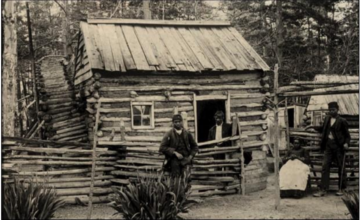
Figure 47. Photograph of a cabin with stick and mud chimney, Bon Air, Virginia, 1888. Note the wooden chimney off the left side of the cabin and the two poles supporting the chimney. Also, note the lack of grass around the cabin, likely indicating the presence of a swept yard. Image from Stottman and Stahlgreen (2017, 9).
