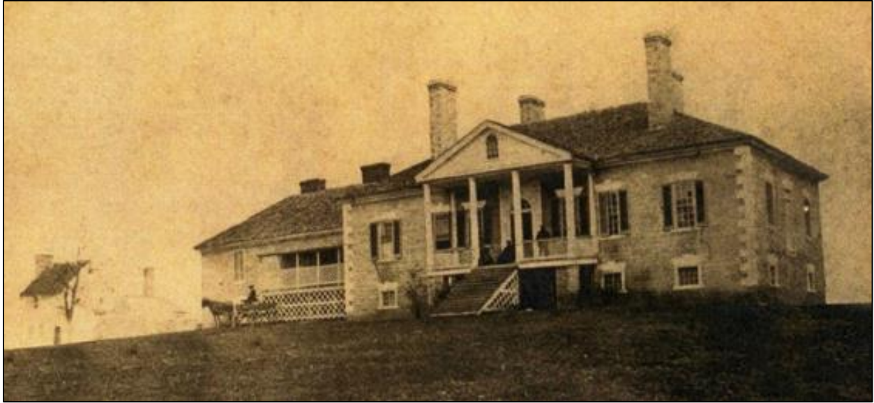
Figure 43. Manor house grounds, 1860s. The manor house is in the center of the image, with Old Hall to the left, and an outbuilding in between the two. The lighter-colored stones at the corners of the manor house and above the windows are the sandstone coining and trim (respectively). Image courtesy of Belle Grove, Inc.
