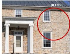
Elsewhere on the building, inappropriate mortars were used to make repairs over the years, causing further harm to the building. Belle Grove had the original mortar analyzed and specially mixed for the repointing project. The building is
